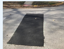
Permanent asphalt patching in the road.
