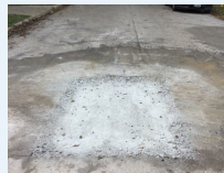
Temporary repair patch in street and/or sidewalk after service line replacement.
