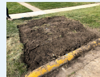
Holes are temporarily backfilled with soil and left to settle.
